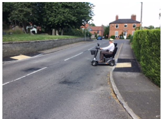
A local resident using the new crossing.
